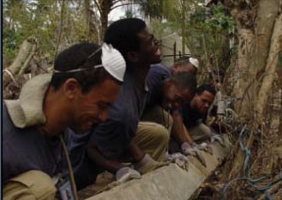
Clearing debris to make way for new homes.
